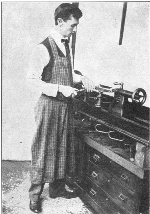
Fig. 237. Position in Roughing Long Piece.
